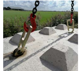
Attach the hooks to the anchors and the load is ready to be lifted
