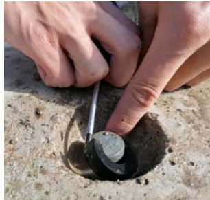
Remove the rubber from the anchor
