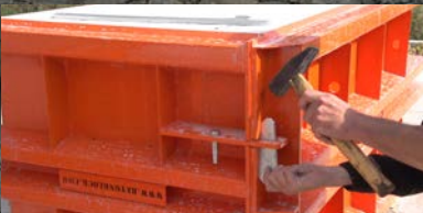
Removing pins and wedges
