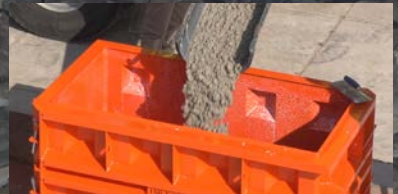
Pouring the concrete
