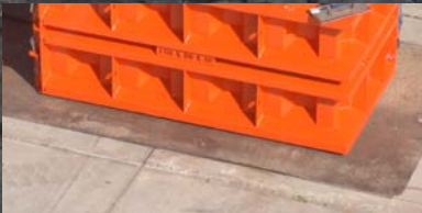
Place mold on leveled surface
